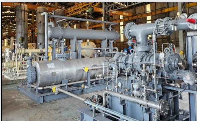
Fabrication is complete on Condor's 1st LNG liquefaction unit
