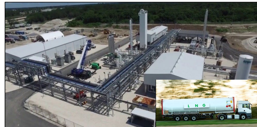
Modular LNG Plant –75,000 Tonnes Per Annum
