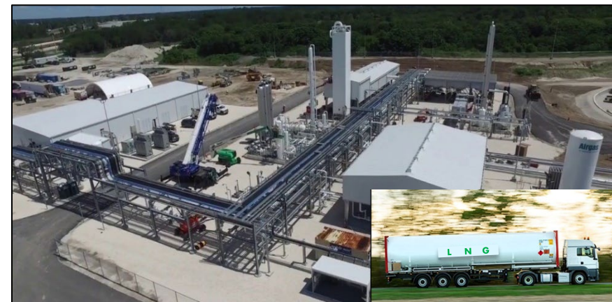
Modular LNG Plant –75,000 Tonnes Per Annum
